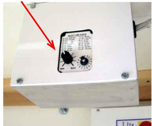
Relay timer adjustment
